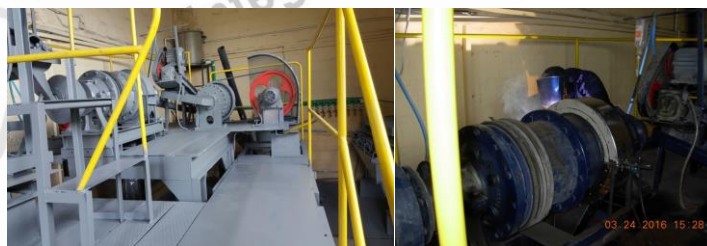
FIGURE 4 - RECONSTRUCTED FLOTATION PILOT PLANT FOR PYRITE CONCENTRATE PRODUCTION AT BOR INSTITUTE
